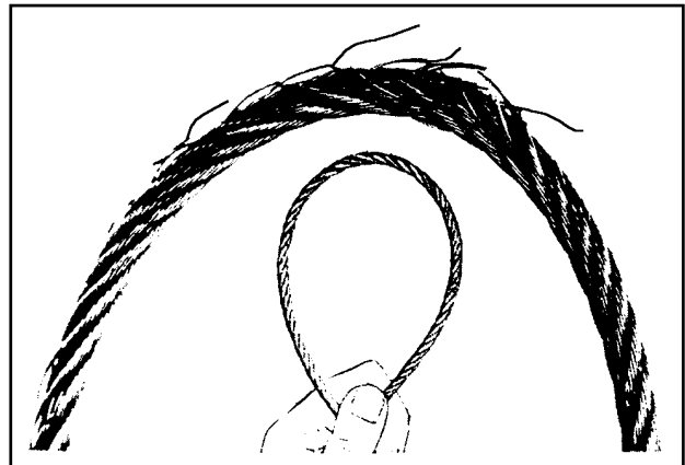
FIGURE 7-16. Cable inspection technique.
